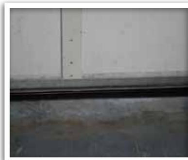
8. Close the garage door to keep constant pressure on the threshold for twenty-four (24) hours.
