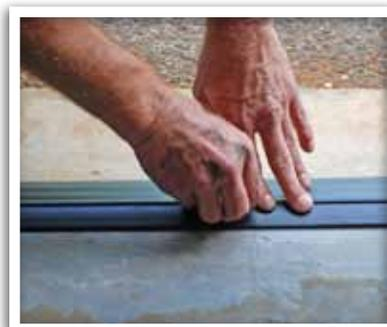
7. Inspect the threshold to make sure it is still between the pencil lines. The position can be slightly adjusted for a short period of time. The length of time varies depending on ambient conditions.
