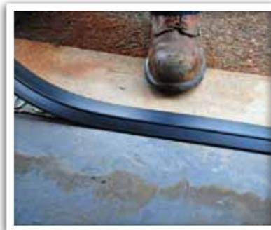
6. Replace the threshold between the pencil lines and firmly press into place. Carefully apply pressure to the threshold to ensure the adhesive spreads uniformly.
