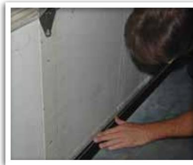
3. With the pencil, mark the inside edge of the threshold on the floor the full length of the threshold (from one door jamb to the other).
