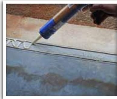
5. Remove the threshold and apply three rows of adhesive the full length of the door between the pencil lines as shown.
