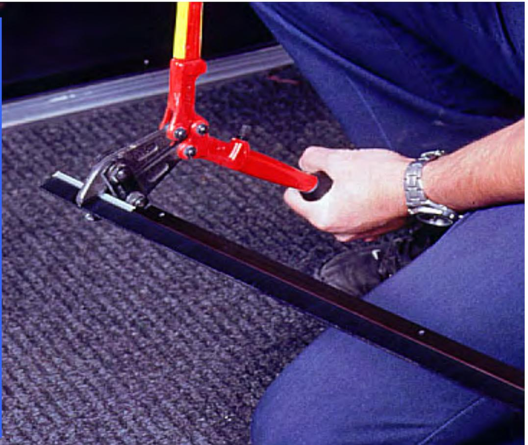
Step 4 - Pry the holder open slightly to allow easy insertion of the brush.
