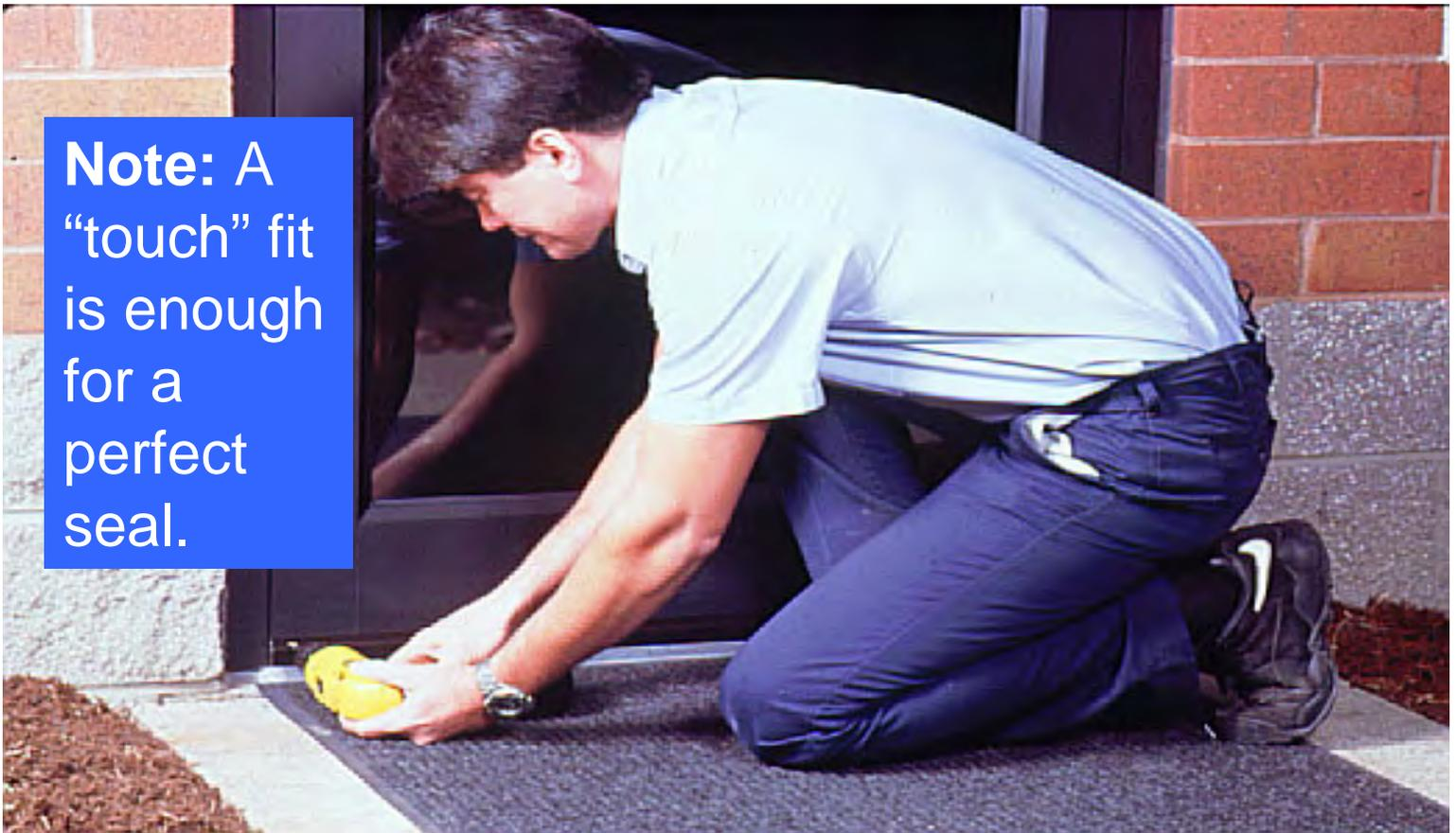
**Installation Instructions for Sealeze Pest Control Door Sweep**
