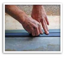
8. Close the garage door to keep constant pressure on the threshold for twenty-four (24) hours. ALLOW AT LEAST 24 HOURS FOR ADHESIVE TO DRY BEFORE
