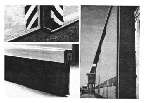
BIG BRUSHOFF. Two years ago, Patuxent Naval Air Station Installed brush seal around the gaps of Its large hangar doors (right and upper left) to reduce heat loss. The weatherstripping consists of flexible nylon bristles (lower left) that won't crack.
